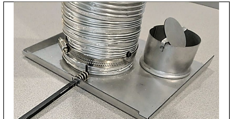
Vent Adapter Flex Connection Hose Clamp first. Secure w/ Screw above Hose Clamp
